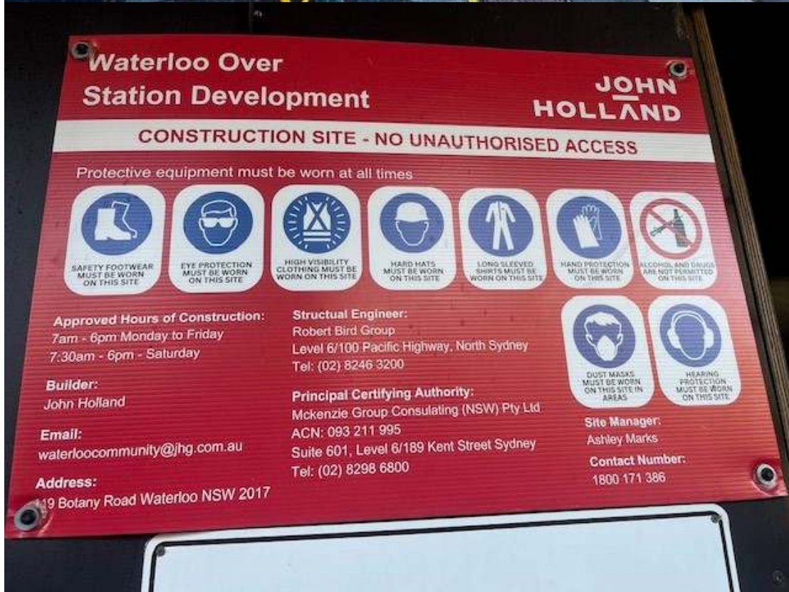
Photos 1-2: Public art was displayed on the hoarding at street level on Botany Road and Wellington Street and included Aboriginal elements and interpretation. Signage was in place as required.
