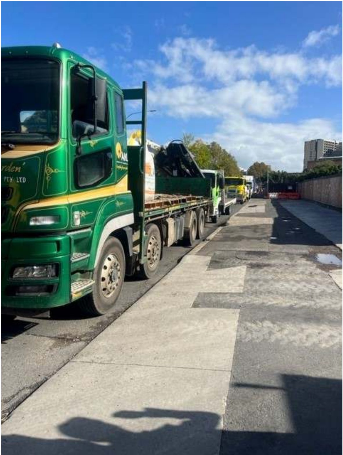
Photo 1: Slip lane in use on Botany Road for loading and unloading during normal construction hours. The slip lane is located within the site boundary so does not require a council work zone approval. There were no significant signs of tracking from the site or the slip lane.
