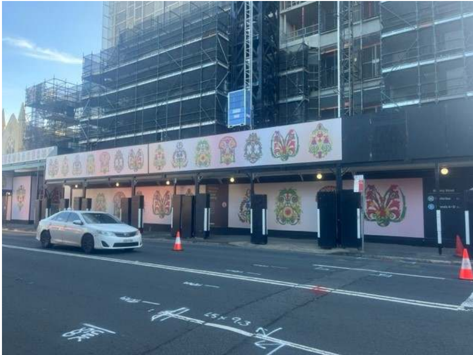
Photos 1-3: Public art was displayed on the hoarding at street level on Botany Road and Wellington Street and included Aboriginal elements and interpretation.
