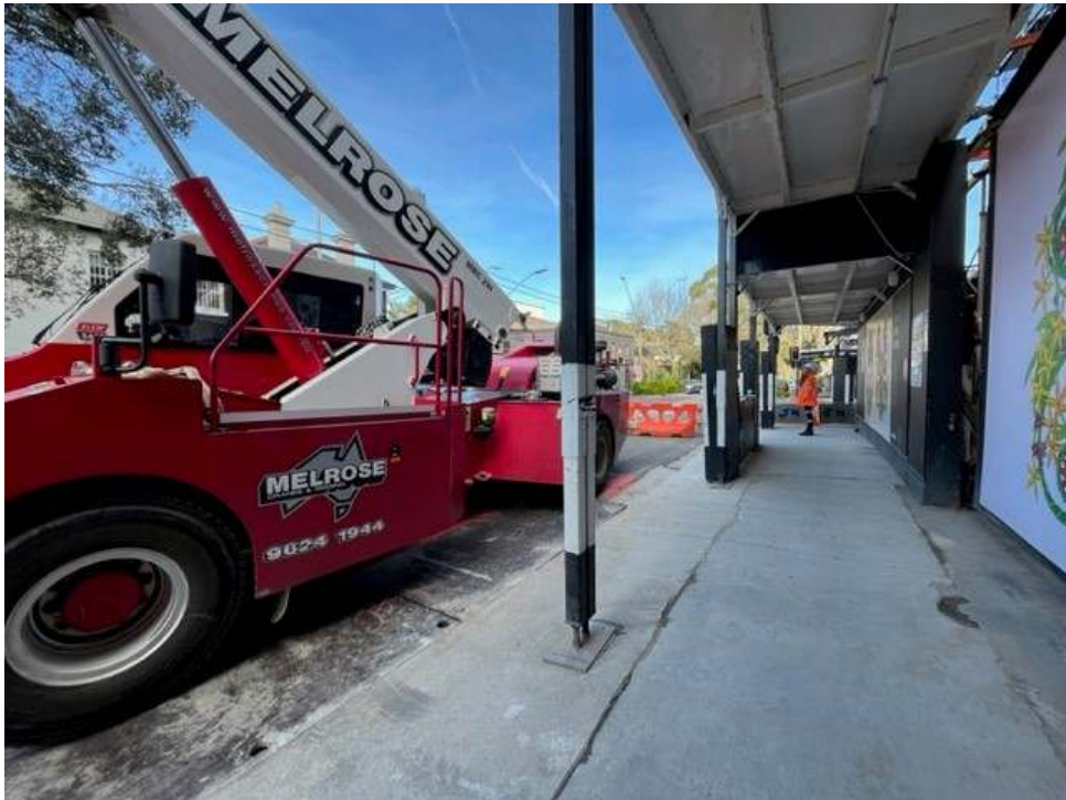
Photo 9: Hoarding and crane on Wellington Street – permits in place as required.
