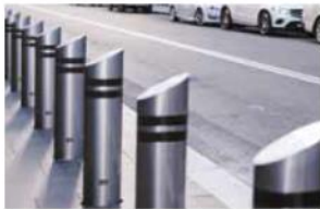
Stainless steel rated bollard
