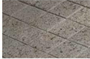
Interlocking concrete unit paver (vehicular grade)
