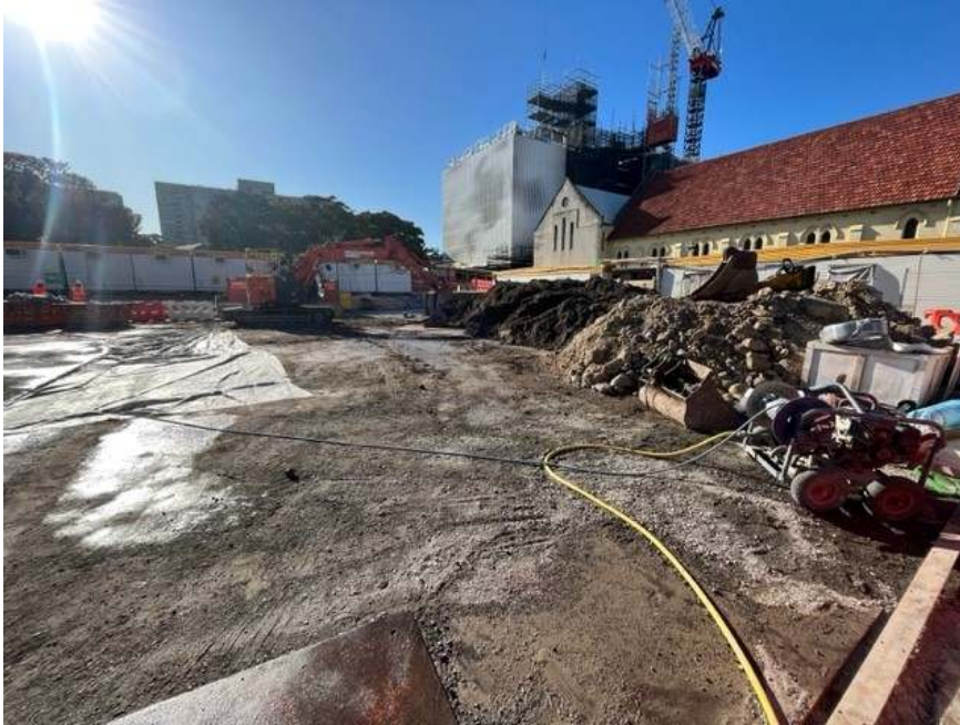
Photo 3: Stockpiling area at the south end of the site
