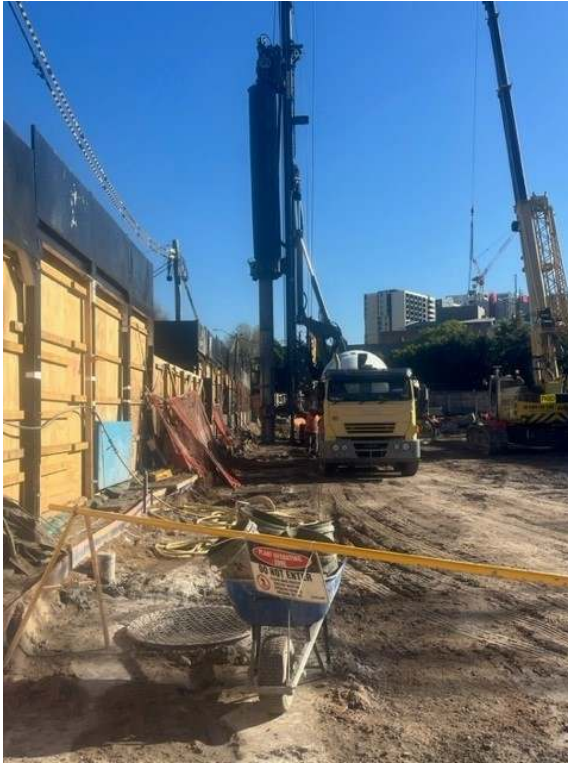
Photo 5: Piling on the western site boundary
