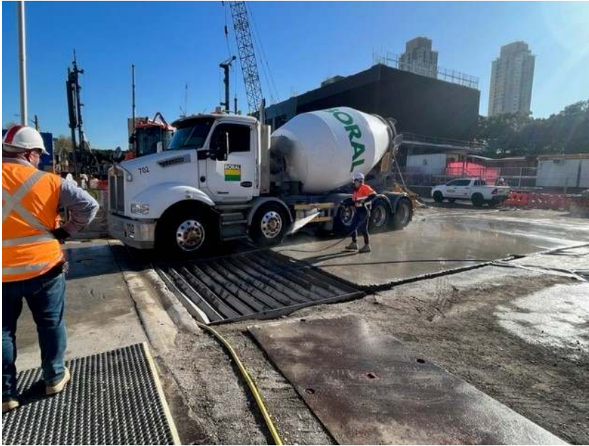
Photo 1: Wheel wash in use for concrete truck exiting the site
