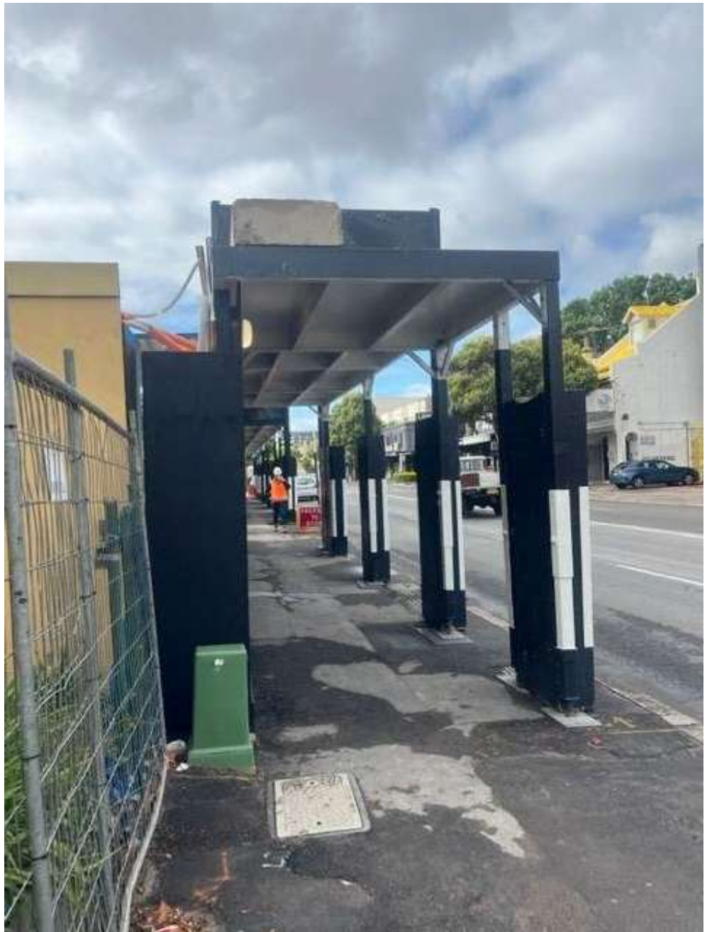
Photo 9: B-Class Hoarding in place along Botany Road
