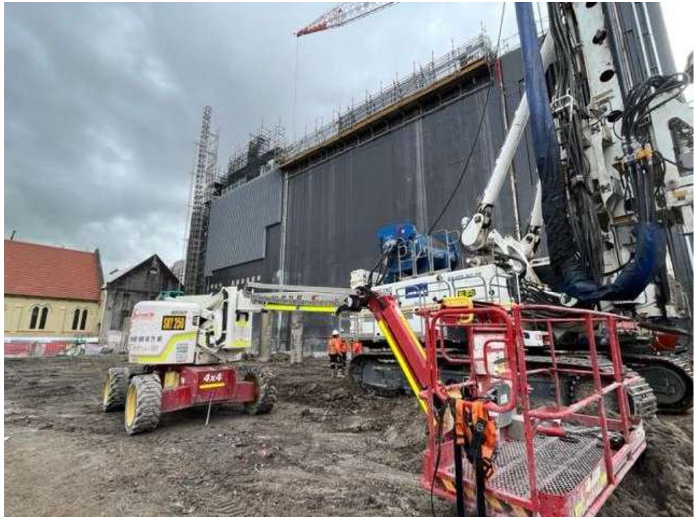
Photo 4: Piling rig and compactor in place on the Southern Precinct site
