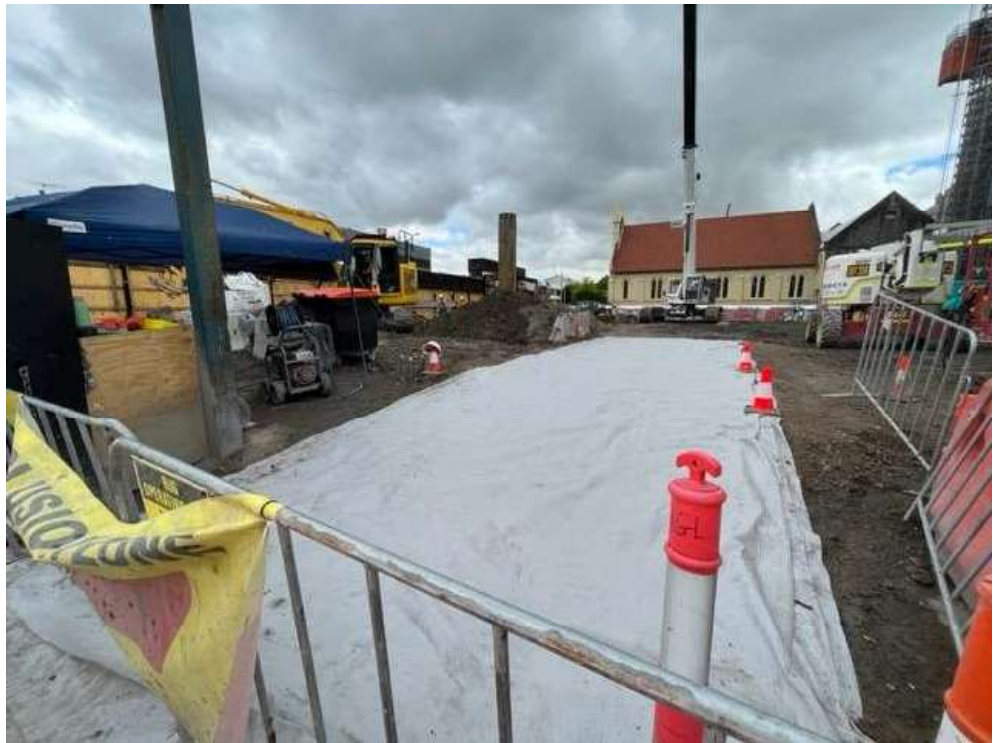
Photo 1: Temporary stabilisation of site access onto Wellington Street
