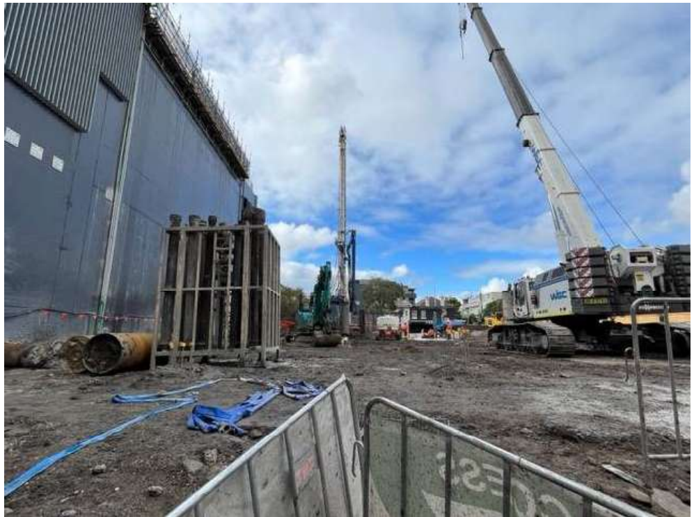
Photo 3: Piling rig and crane in place on the Southern Precinct site
